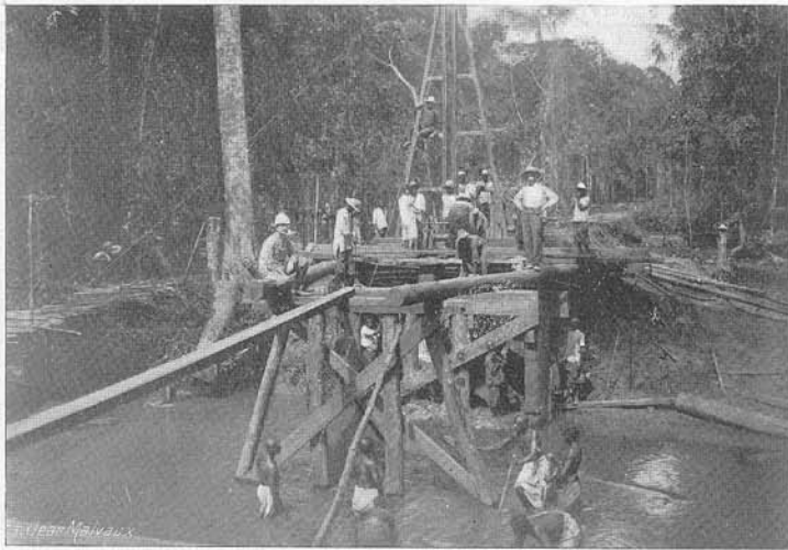
Temporary Bridge in course of erection
