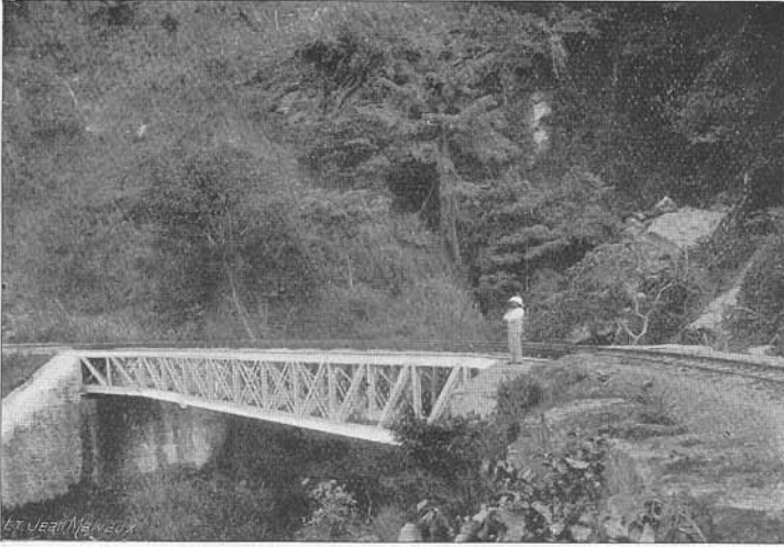
A Bridge on the Railway
